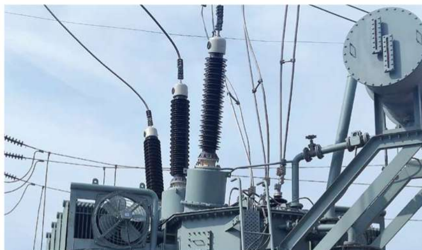
Yash make 145kV OIP bushings on a 100 MVA power transformer
